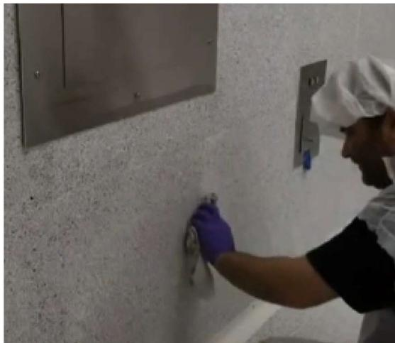
Photo #4: Remove excess caulking compound
