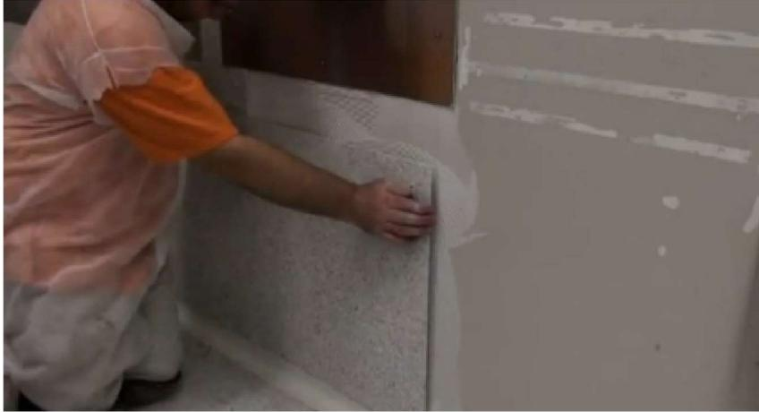
Photo #1: Placing tile into adhesive on wall.
