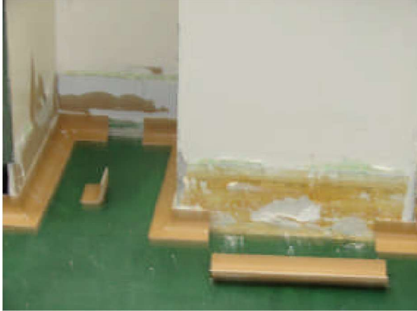
Photo #1: Cut sanitary base to fit
