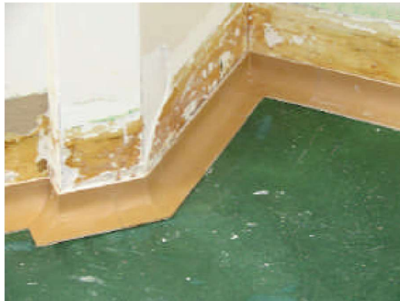
Photo #3: Finished sanitary base
