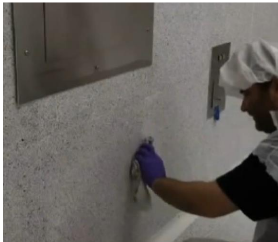
Photo #4: Remove excess caulking compound
