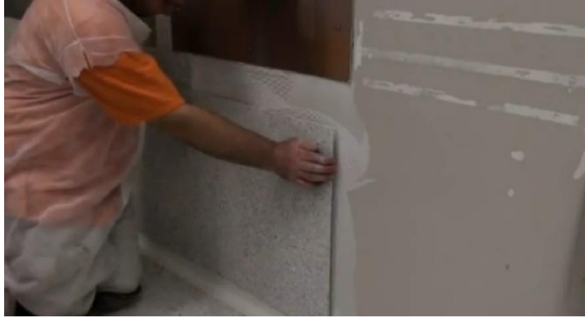
Photo #1: Placing tile into adhesive on wall.
