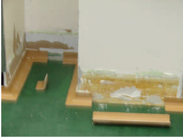
Photo #1: Cut sanitary base to fit
