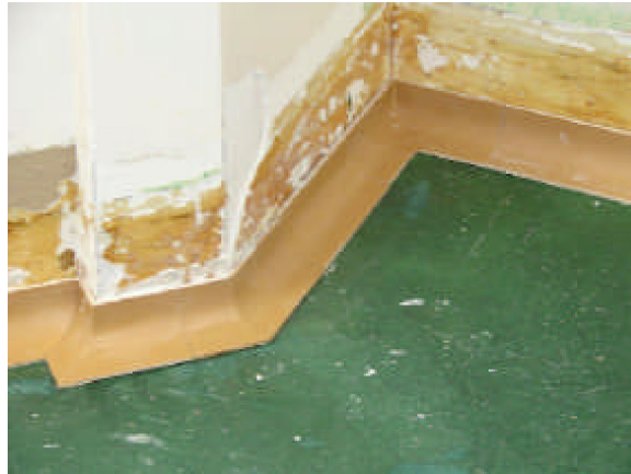
Photo #3: Finished sanitary base
