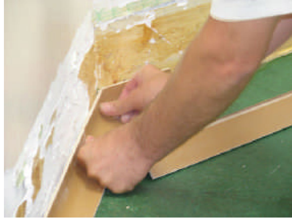
Photo #2: Secure base with adhesive
