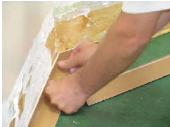
Photo #2: Secure base with adhesive
