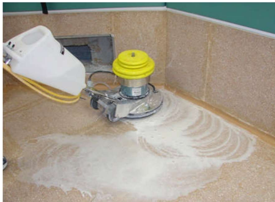
Wet-polishing procedure to remove any residue and eliminate lippage.
