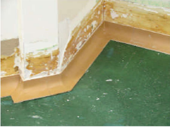
Photo #3: Finished sanitary base
