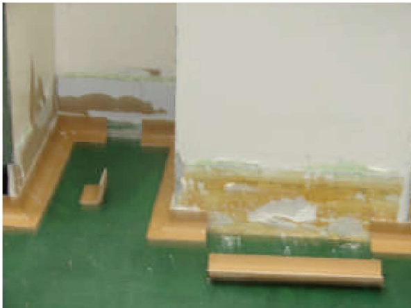
Photo #1: Cut sanitary base to fit
